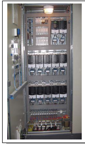
INVERTER CABINET ROLLER CONVEYORS SPEED CONTROL
